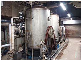
Example of reuse of wastewater: Water filtration system at Shinjuku Washington Hotel Honkan
