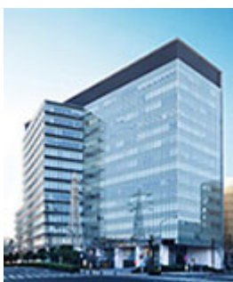
B37 ARENA TOWER
