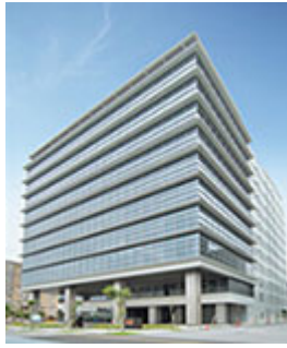
E3 Tsubokawa Square Building
