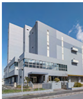
E15 Hirakata Nagao Logistics Center
