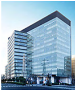
B37 ARENA TOWER
