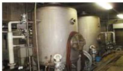
Example of reuse of wastewater: Water filtration system at Shinjuku Washington Hotel Honkan
